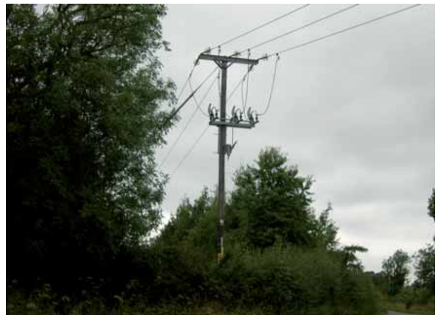
3. A typical 11kV overhead line.
