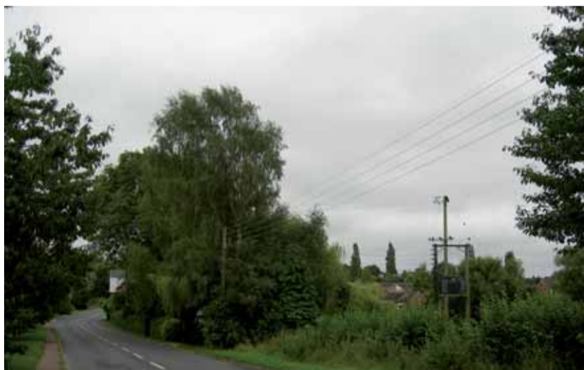
1. LV showing the typical four-bare-wire-conductor construction.
