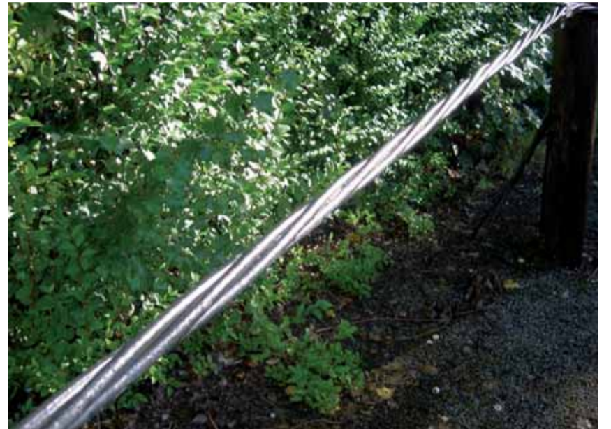
2. Close-up of the ABC construction.
