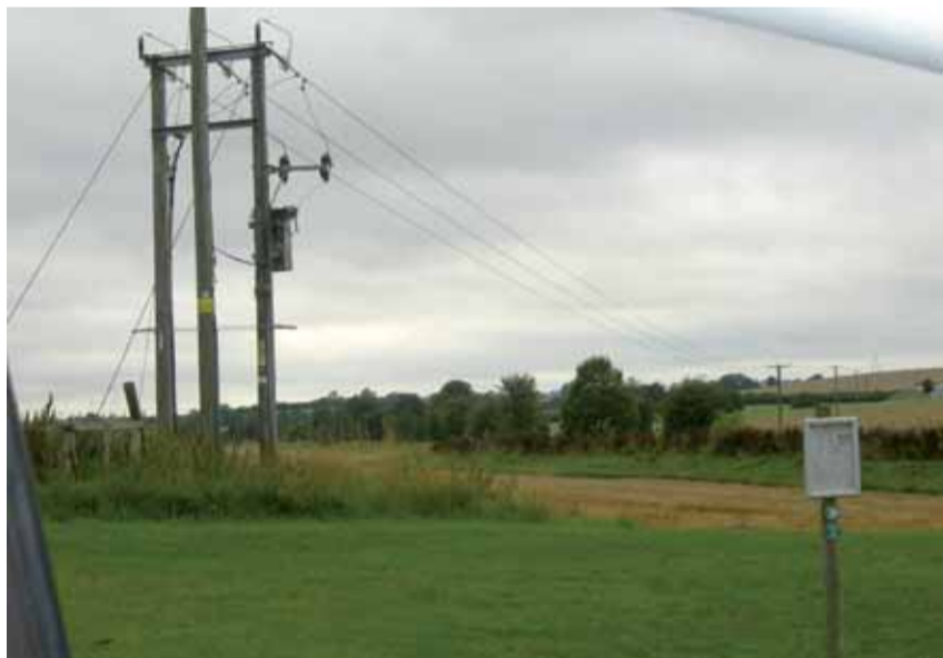
5. A typical 33kV overhead line.
