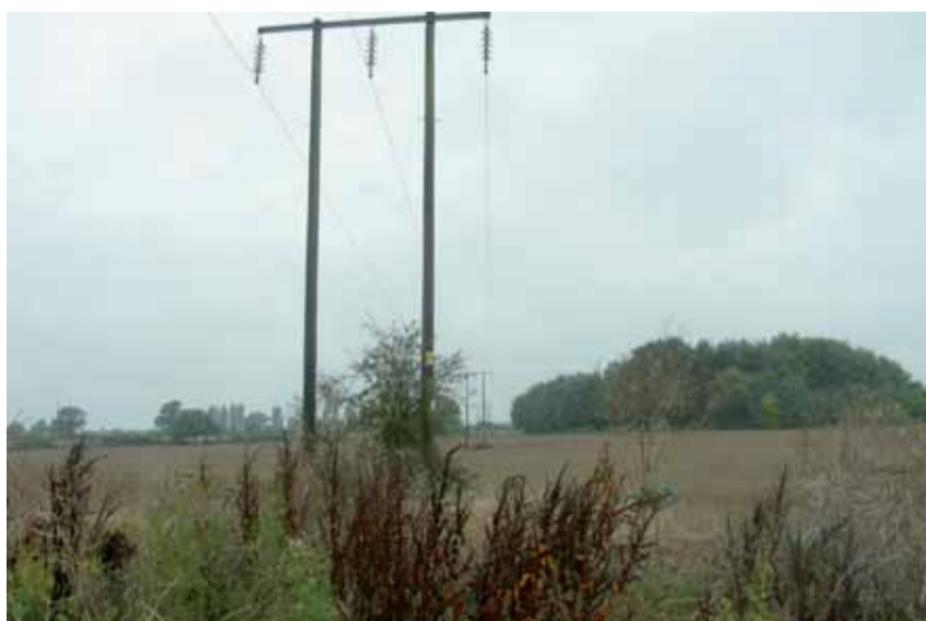
6. A typical 66kV overhead line.
