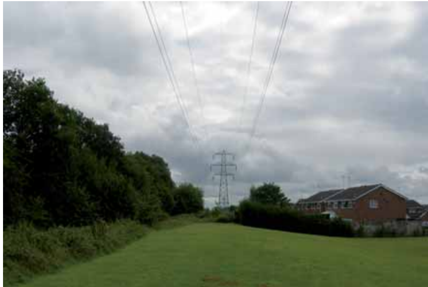
4. A typical 132kV overhead line.
